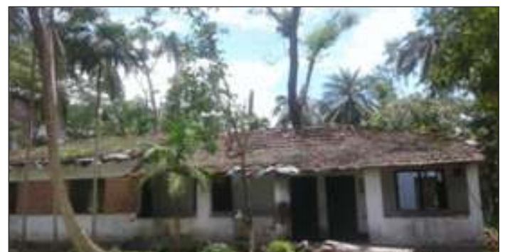
Damaged School Building
