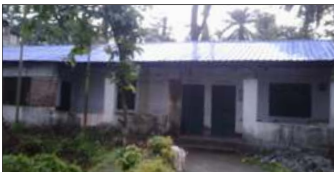
Renovated School Building
